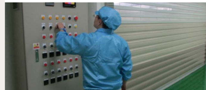
Complete in-house Qualification Control
